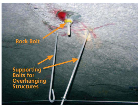
Figure 1. Rock bolts and supporting bolts commonly used in underground space
