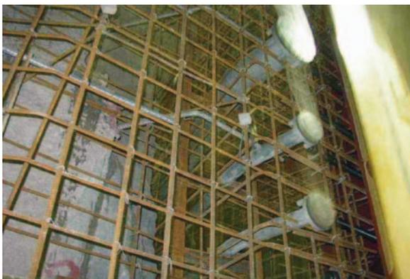
Figure 6. Equi-potential bonding of metallic services at entry points before concrete walls are cast
