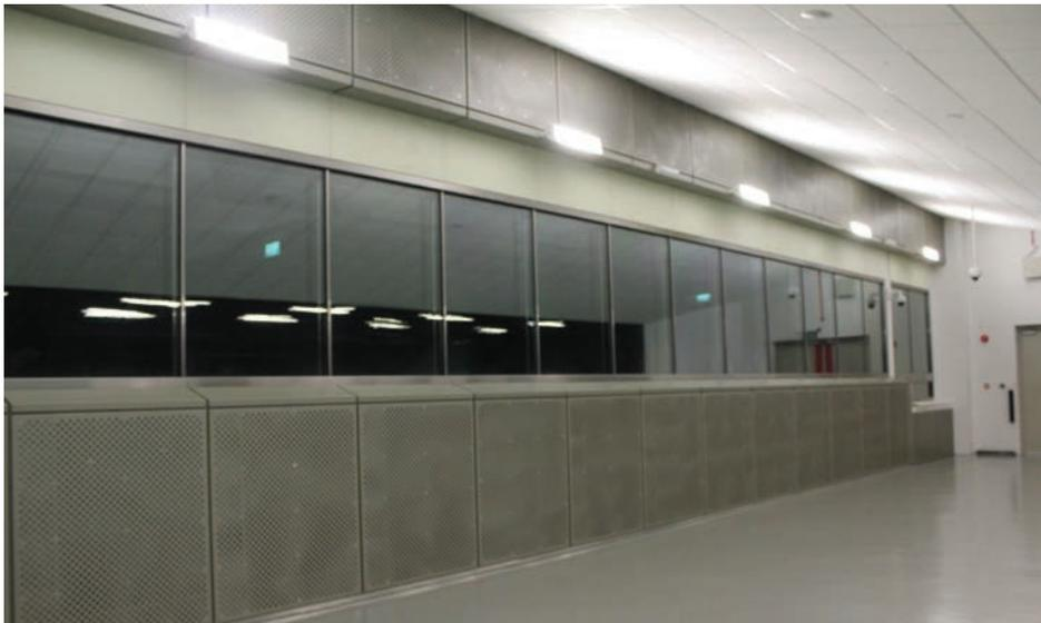
Figure 12. Ballistic glass installed at the control room and learning gallery
