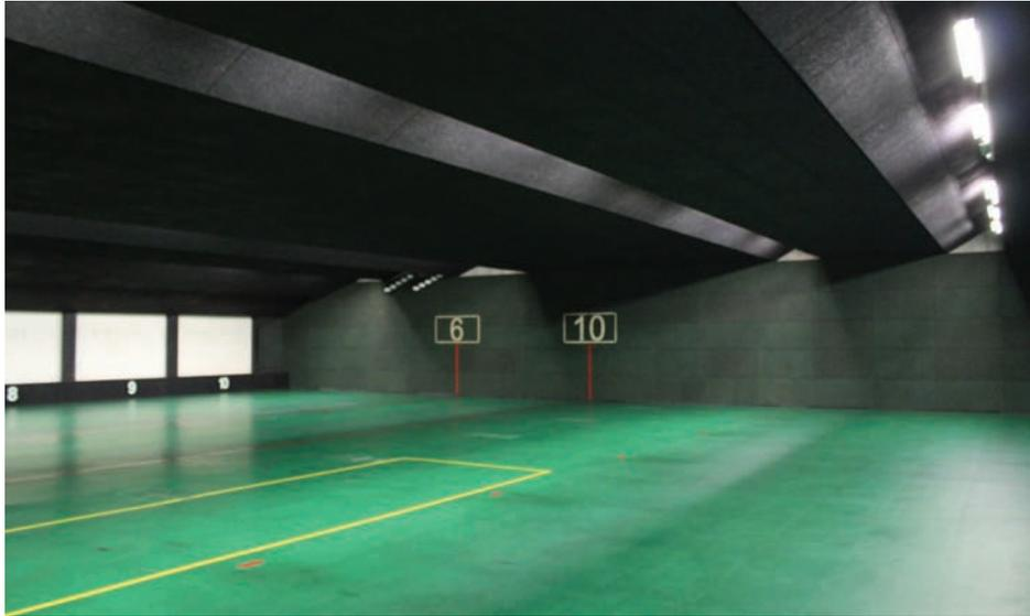
Figure 10. Ceiling baffles in 50m Range 1 and 2
