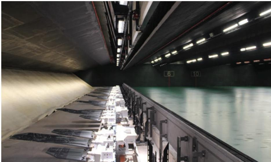
Figure 11. Redirective guards used at the bullet traps
